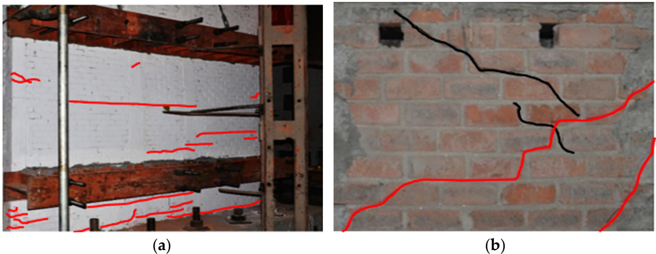
Figure 13. Cracking patterns on the surface of transverse wall and inner longitudinal wall. (note: Cracks generated by the application of thrust are marked with black symbols, whereas those generated by the application of tensile force are marked with red symbols. (a) Cracks on the transverse wall. (b) Cracks on the interior longitudinal wall.
