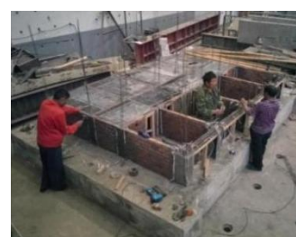
(c) Masonry walls at ground-level floor
