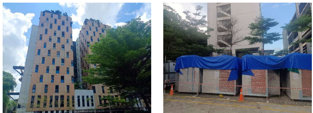
Figure 1. On-site MRU construction environment (left) and the controlled assembly environment at the Singapore factory (right).
