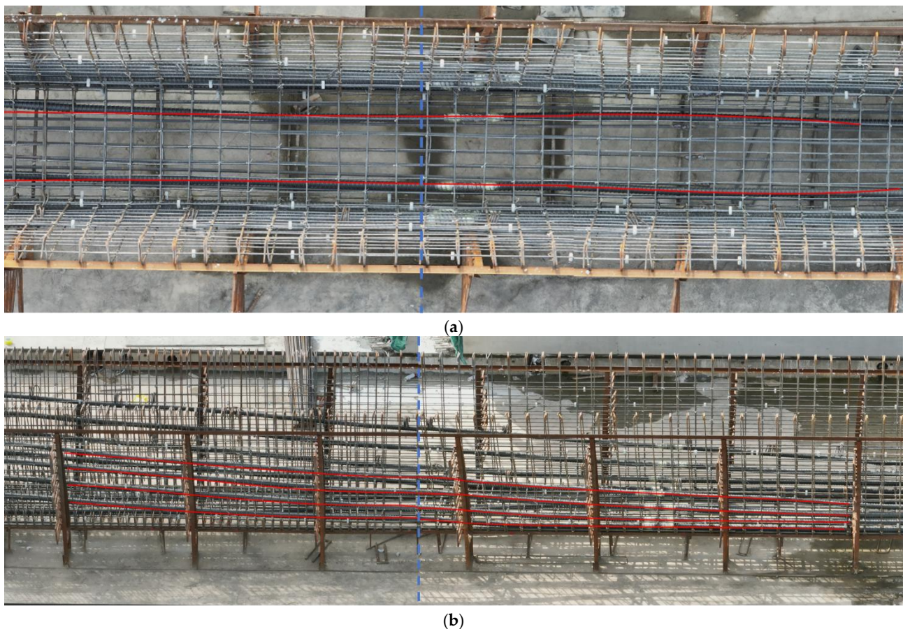
Figure 8. Image Stitching Result: (a) Overhead. (b) Front view.
