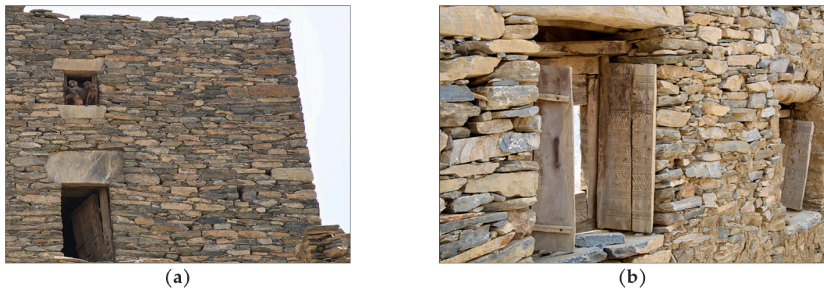
Figure 6. Openings and thresholds as customary governance evidence: (a) limited door and window openings in a load-bearing madameek wall; (b) threshold and timber joinery detail. Source: Author field documentation, 2014.
