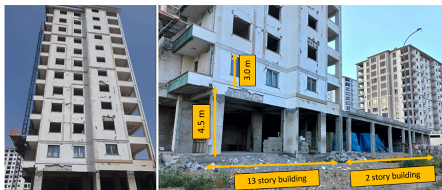
Figure 5. Investigated multi-story building.
