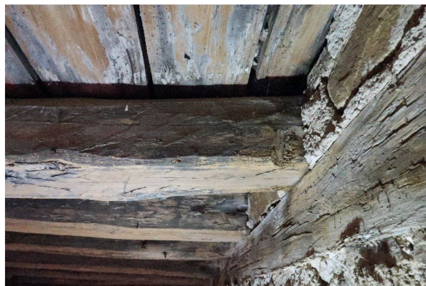
Figure 3. Sleepers embedded in the masonry.
