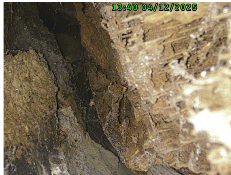
Figure 14. Example of endoscopy measurement results of the beam no. 7 northern end denoted as position 7.3.4 in Figure 12.
