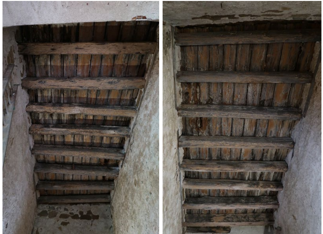
Figure 2. Eastern (left) and western (right) view of the ceiling structure.
