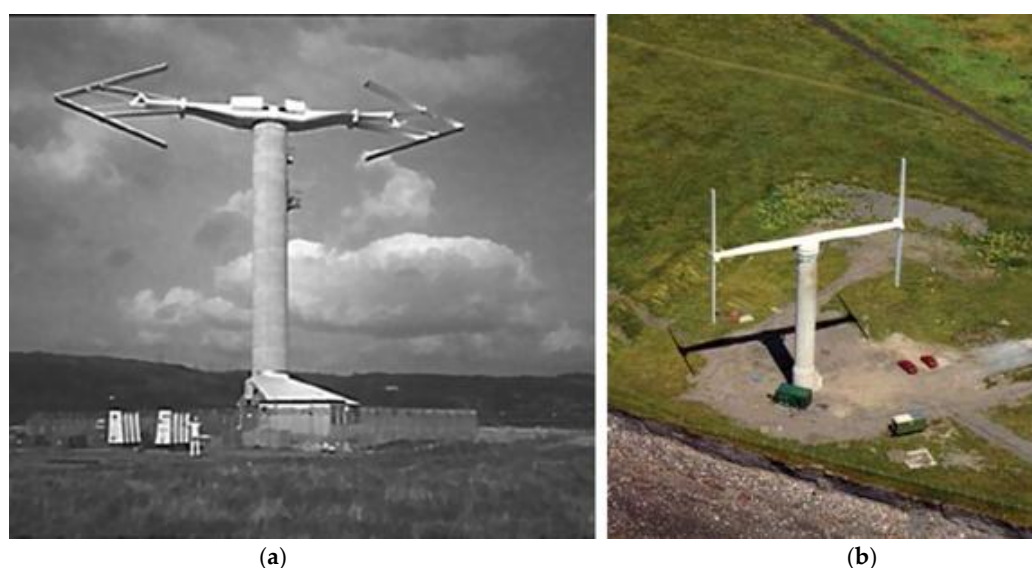
Figure 11. (a) Musgrove turbine in reefed configuration and (b) Musgrove VAWT 850–500. [49]
