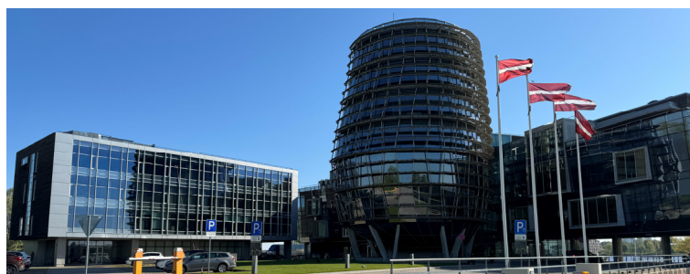
Figure 1. The office building complex examined in the case study (author photo).
