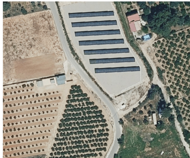
Figure 3. Example of an orange farm transformed into a solar park in the Valencia region (source Google maps).
