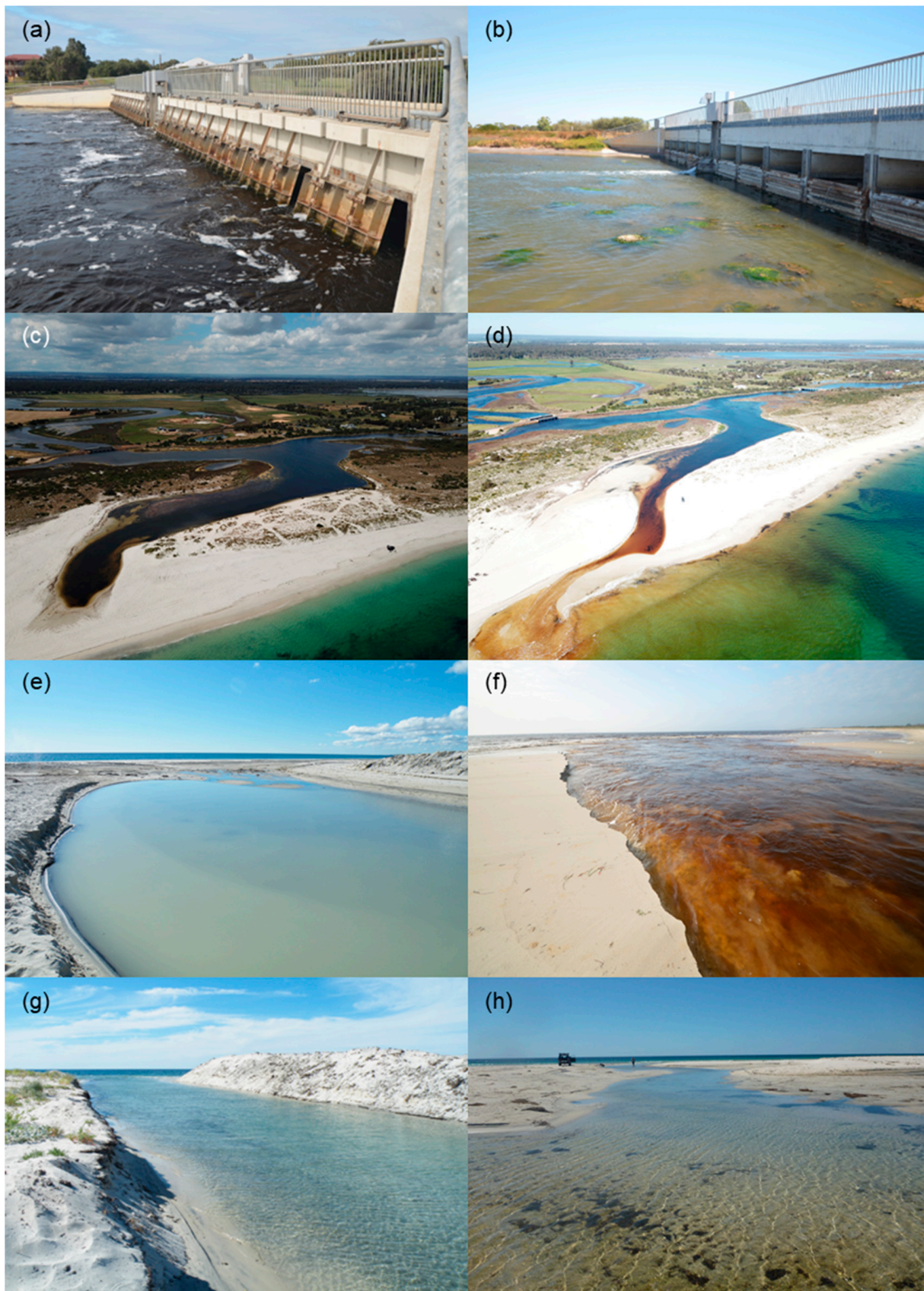
Figure A1. Photographs showing (a) the downstream side of the Vasse surge barrier during winter when freshwater discharge was sufficient to open the flap gates and (b) the stop boards installed on the upstream side of the Wonnerup surge barrier in summer. Drone photographs of the sand bar in Wonnerup Inlet when (c) closed and (d) open to the ocean. Photographs of the bar in four of the major hydrodynamic phases described by Whitfield et al. [13], i.e., (e) closed, (f) outflow, (g) tidal and (h) semi-closed. Note the sediment being scoured away in (f) and the pile of sediment deposited from the mechanical breaching in (g). Photographs (a,b,d–h) were taken by James Tweedley and (c) by Kurt Krispyn.
