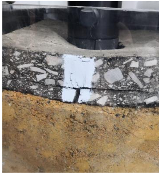
Figure 11. Failure mechanism after testing the specimen with the granular base as a support.
