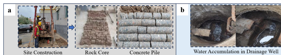
Figure 3. On-site exploration and research: (a) core sampling; (b) utility survey.
