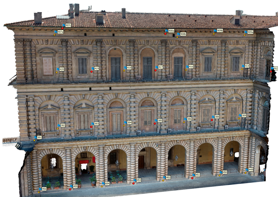
Figure 5. South-west façade of the courtyard of Palazzo Pitti with CPs (yellow dots) and ChPs (red dots).
