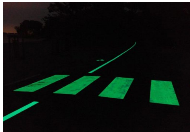
Figure 4. Luminescent road markings (Source: [24]).
