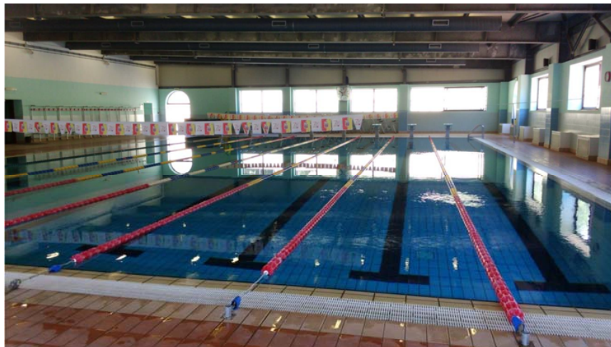
Figure 1. Indoor swimming pool.
