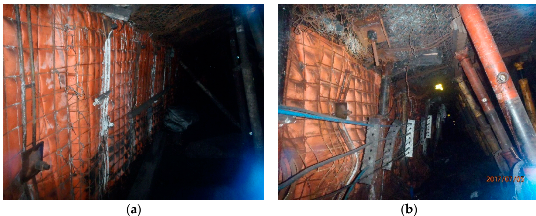
Figure 15. Comparison of the deformation of the gob-side retaining entry with and without shallow hole blasting: (a) with shallow-hole blasting; (b) without shallow-hole blasting.
