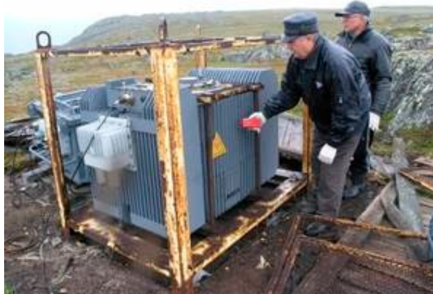
Figure 6. Radioisotope Thermoelectric Generator (RTG) used to supply power to lighthouses and navigation beacons [106].
