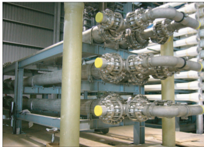
Figure 6. Rack design of a triple DWEER™ [13].
