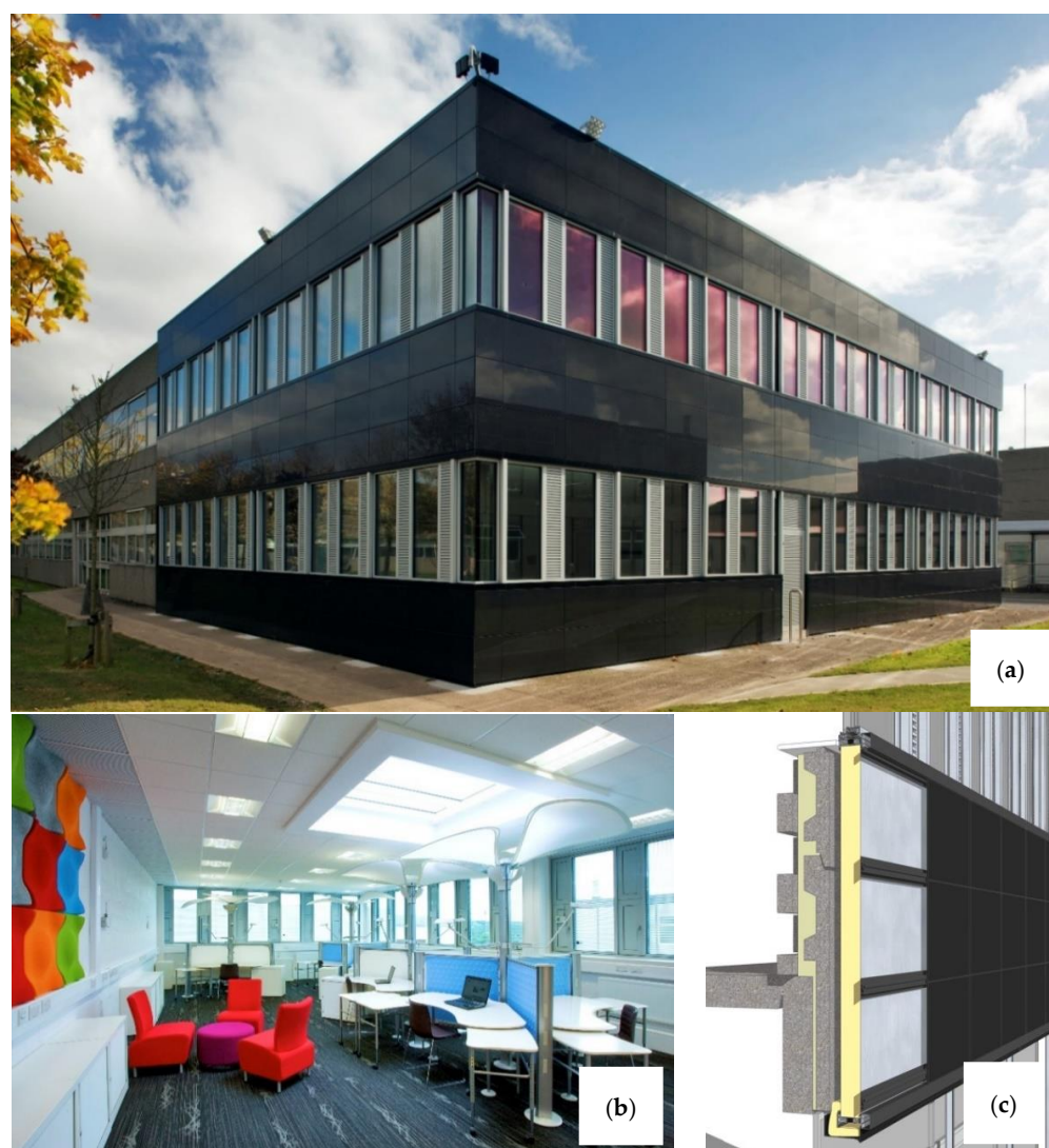
Figure 1. NBERT in the zero2020 building: (a) image of exterior of retrofitted building; (b) image of open plan office with MCSL ventilation system; (c) image of high-performance retrofitted wall detail.
