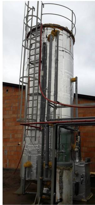
**Figure 8.** Monosubstrate flow reactor for methane fermentation of slurry with a biogas production installation-view (photo by Grzegorz Wałowski).
