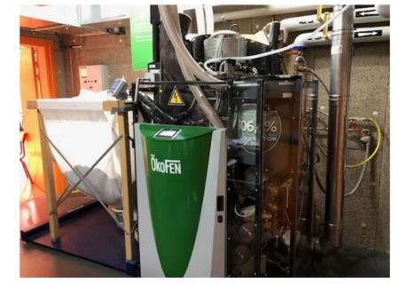
Figure 5. Micro-CHP unit installed in laboratory@ Paris Nanterre University.
