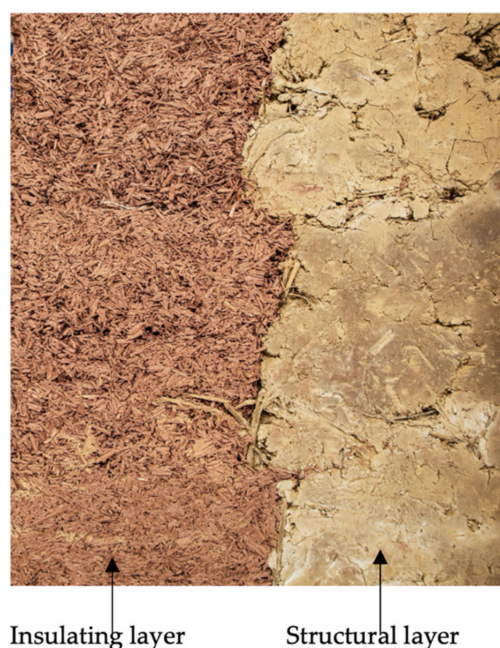
Figure 1. Photo of cob composite wall.
