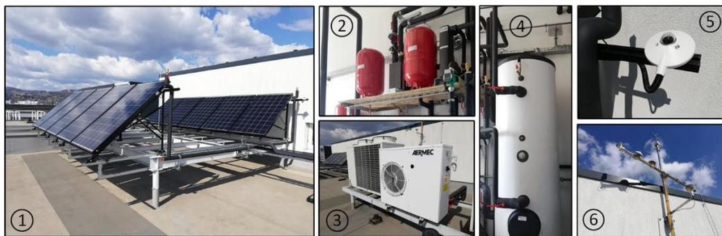
Figure 2. PV/T system: (1) PV/T modules, (2) heat exchangers, (3) refrigeration unit, (4) TEST, (5) pyranometer, and (6) anemometer and ambient temperature sensor.
