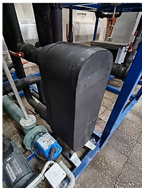
Figure 3. The plate evaporator positioning in the system. Source: own elaboration.
