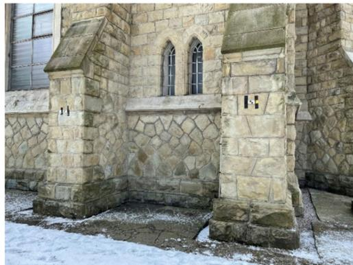
**Figure 3.** Fixing the warp points on the church buttresses.
