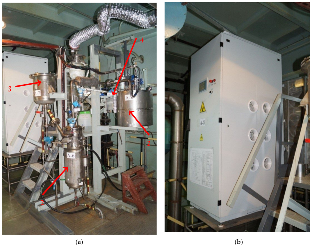
Figure 2. General view of the installation: (a) 1, the resonator chamber with the crucible; 2, the bubbler; 3, the dispensing vessel; 4, the waveguide) and (b) the magnetron control box.
