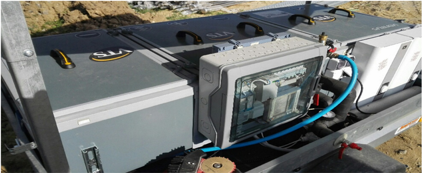
Figure 3. View of the PC FCH HVAC 1700 air handling unit. Source: the authors.
