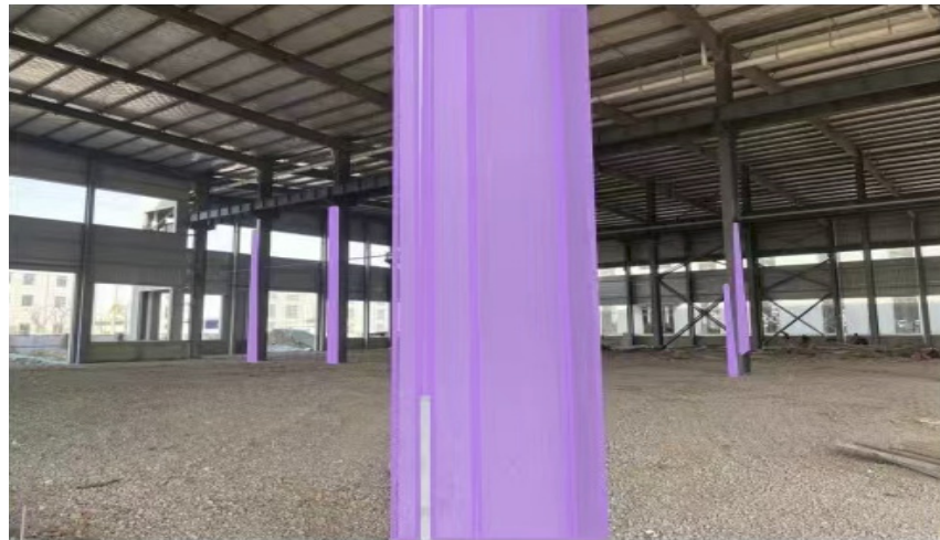
Figure 16. Preliminary segmentation results of steel structure columns.
