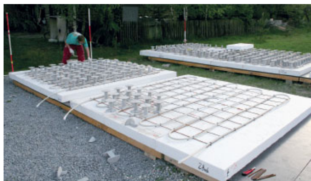
Figure 3. Use of active thermal protection in the reinforced concrete core of the building envelope as a thermal barrier concreted directly in-site using EPS lost formwork (source: ISOMAX) [3].
