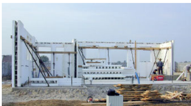
Figure 3. Use of active thermal protection in the reinforced concrete core of the building envelope as a thermal barrier concreted directly in-site using EPS lost formwork (source: ISOMAX) [3].
