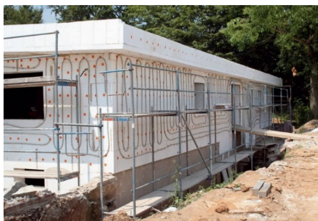
Figure 2. Application of active thermal protection as a thermal barrier on the exterior side for the application of heat from the unfrozen depth of the ground (source: ISOMAX) [3].
