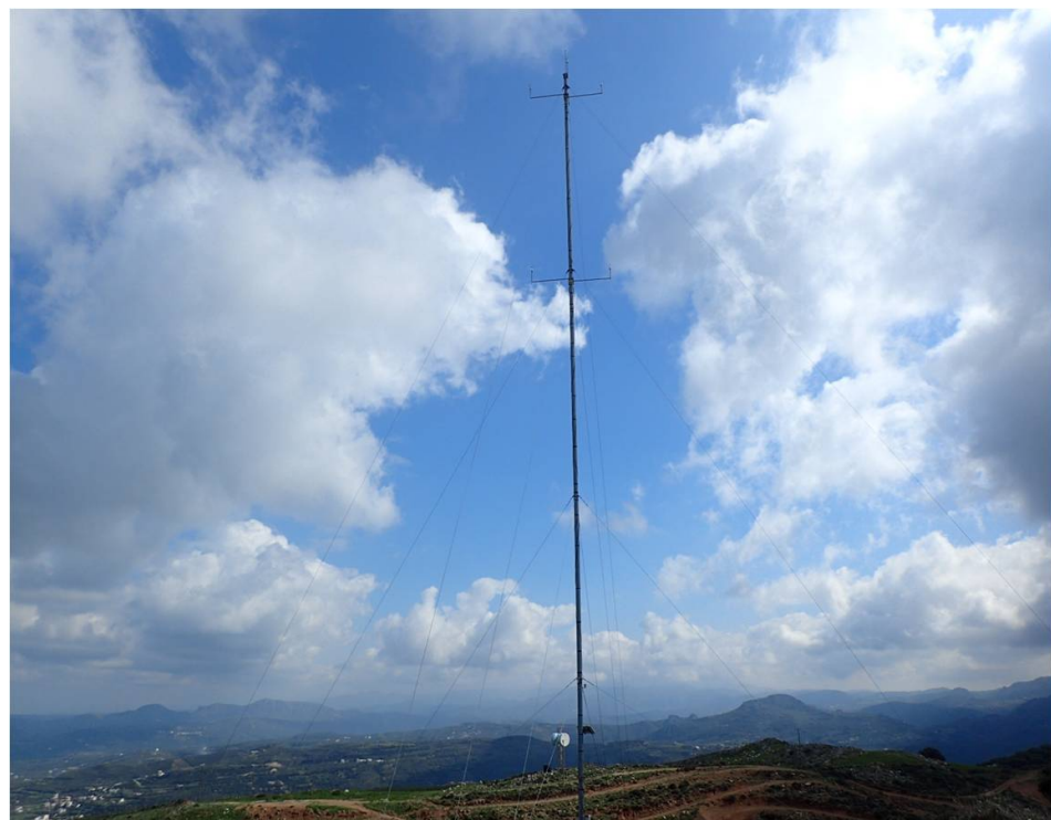
Figure 2. Photograph of the 30 m meteorological mast and its surrounding area at Toplou.
