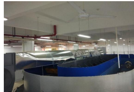
(b) Side view of the water tank.
