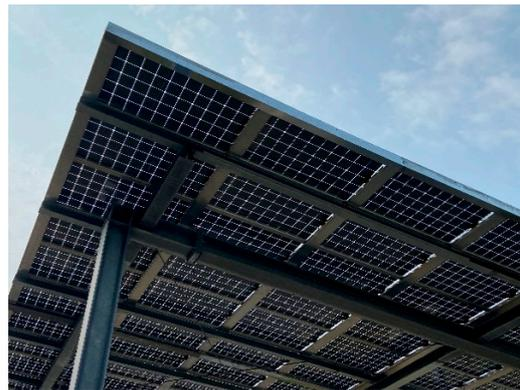
**Figure 15.** Final PV-SÜD demonstrator at the Hegau site, with the view from below showing the overhead proof of glass-glass PV modules with the dedicated water draining supporting structure @AIT.
