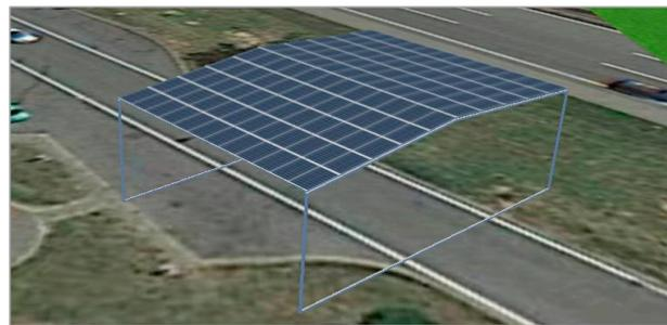
**Figure 10.** PV-SÜD demonstrator at the Hegau site: The roof-type variant is the gable roof.
