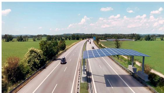
**Figure 5.** Visualization of the gable roof variant.
