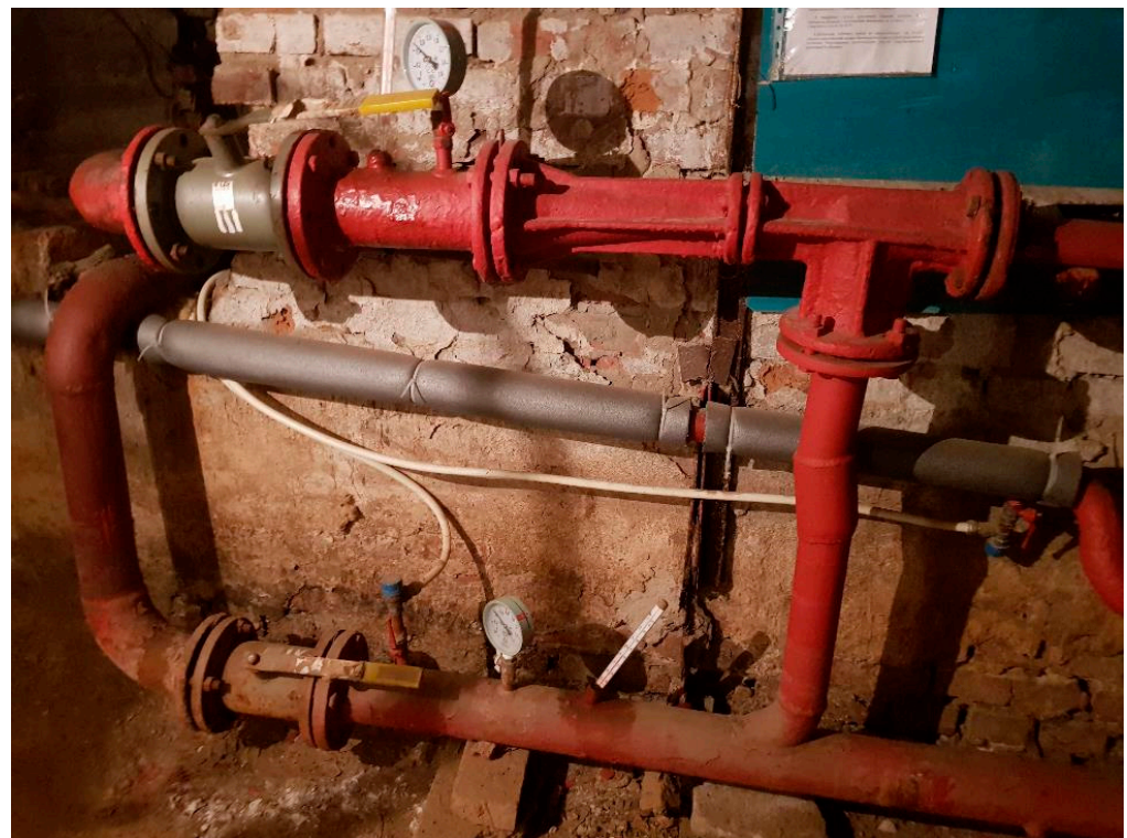
Figure 5. DH substation with a hydroelevator installed; no hydraulic pump is required.
