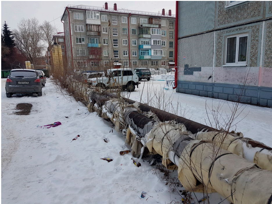
Figure 10. A section of an aboveground DH network characterized by the poor condition of heat insulation.
