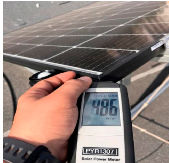
Figure 14. Solar irradiance measurement on the tilted plane using a PYR1307 pyranometer.
