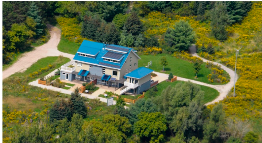
Figure 3. Archetype Sustainable House test facility used as the case study basis for the calibrated model.
