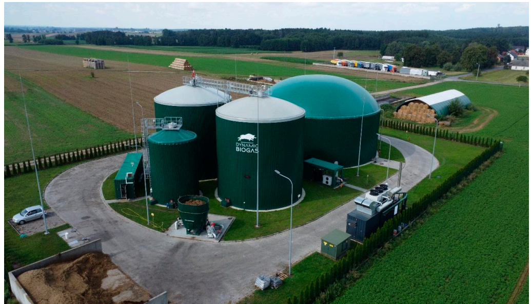
Figure 1. Śniaty agricultural biogas plant (499 kW of electric power) (source: Dynamic Biogas Energy company).
