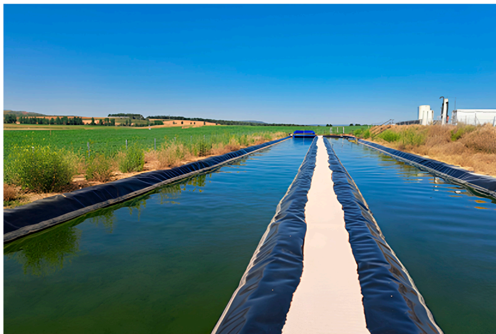
Figure 2. Open raceway pond for microalgae cultivation, showing the circulation paddle and the digestate discharge tube.
