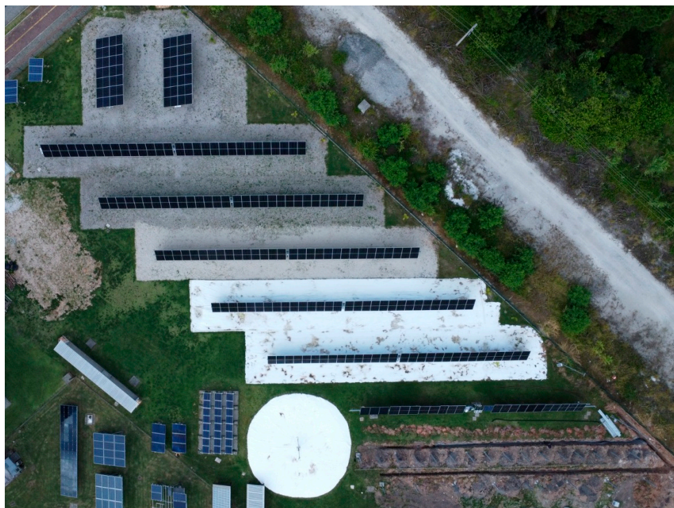
Figure 12. Pilot solar PV plant at the Solar Energy Research Laboratory Fotovoltaica/UFSC in Florianópolis, Brazil (27.4° S, 48.4° W, www.fotovoltica.ufsc.br ), and the albedo station, during the first experimental cycle before cleaning the covers, showing considerable soiling accumulation on the white and pearl-white reflective films due to adjacent construction activities, visible in the lower part of the image.
