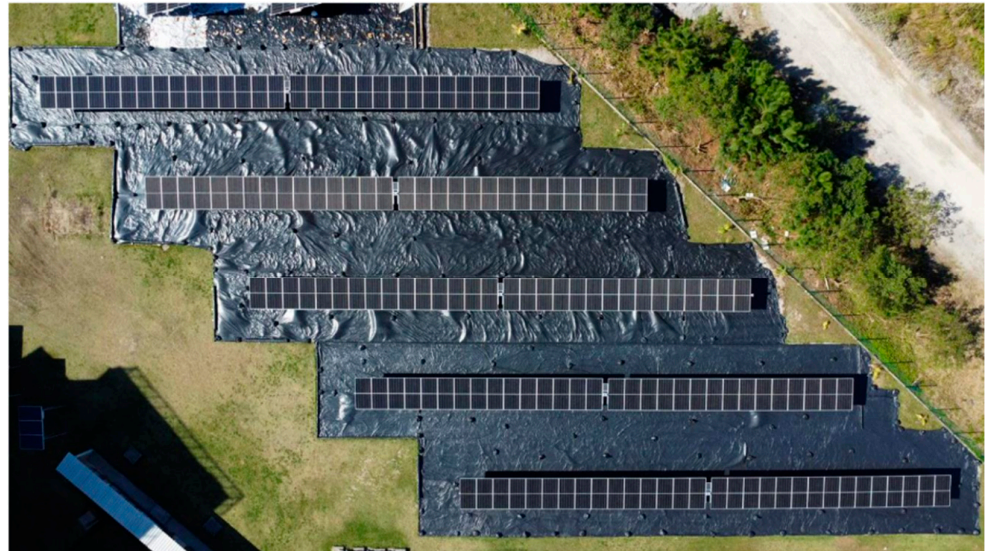
Figure 3. Pilot plant during the baseline period, with black tarps installed below the identical PV systems to homogenize the ground reflectivity and impose a uniform low-albedo condition before the evaluation of the reflective covers.
