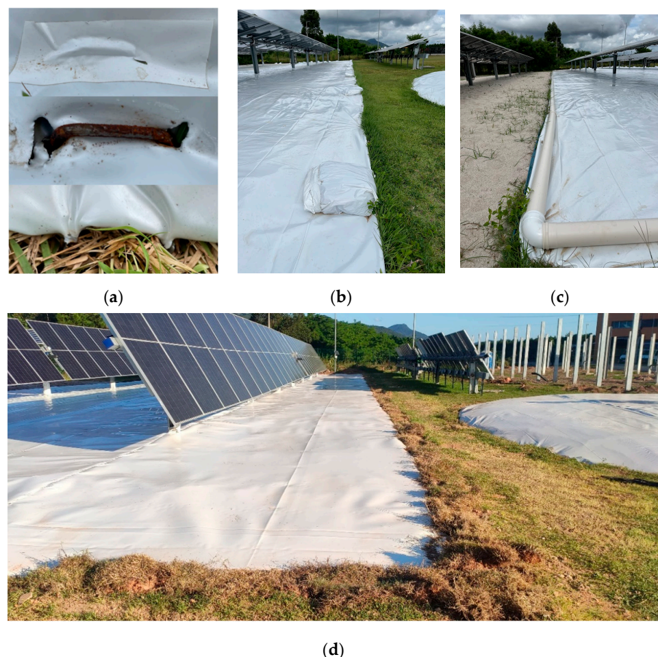
Figure 15. Fixation methods evaluated for the reflective films during the experimental campaign: (a) metallic staples; (b) raffia bags filled with sand; (c) PVC tubes filled with sand; and (d) trench anchoring.
