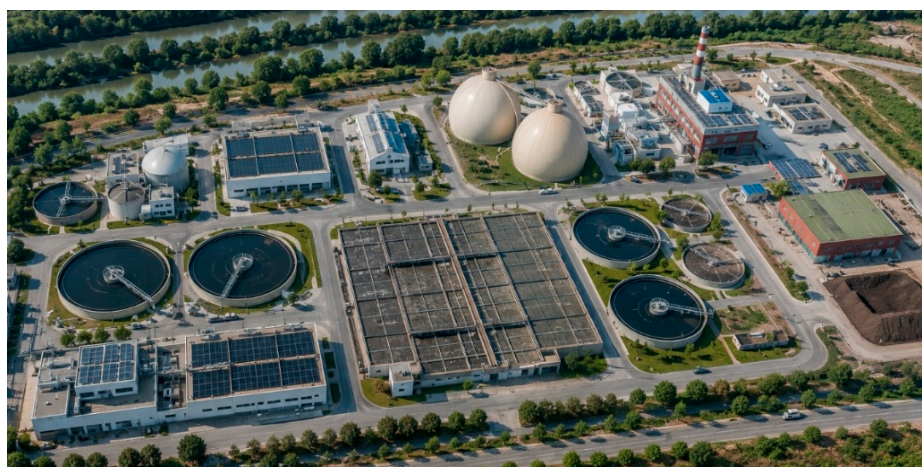
Figure 1. Aerial view of Biofactoría Sur (Granada, Spain), the full-scale municipal WWTTP used in this study.
