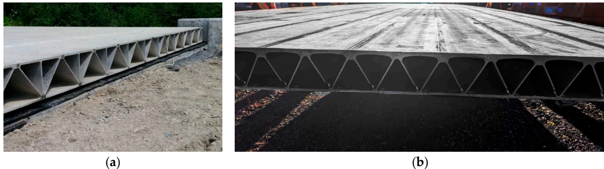
Figure 1. Aluminium bridge decks: (a) Friction Stir Welding (FSW) [8]; (b) Gas Metal Arc Welding (GMAW).
