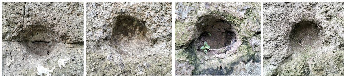
Figure 1. Ballistic marks on stone ashlars in the northern city walls near Vesuvio Gate.
