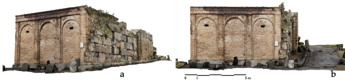
Figure 5. 3D digital model of the remains of Vesuvio Gate and the Castellum Aquae : (a) Perspective view; (b) Orthographic view. Here, the pronounced slope of the cobblestone road, which once led out of Pompeii through the northern gate, is clearly visible.
