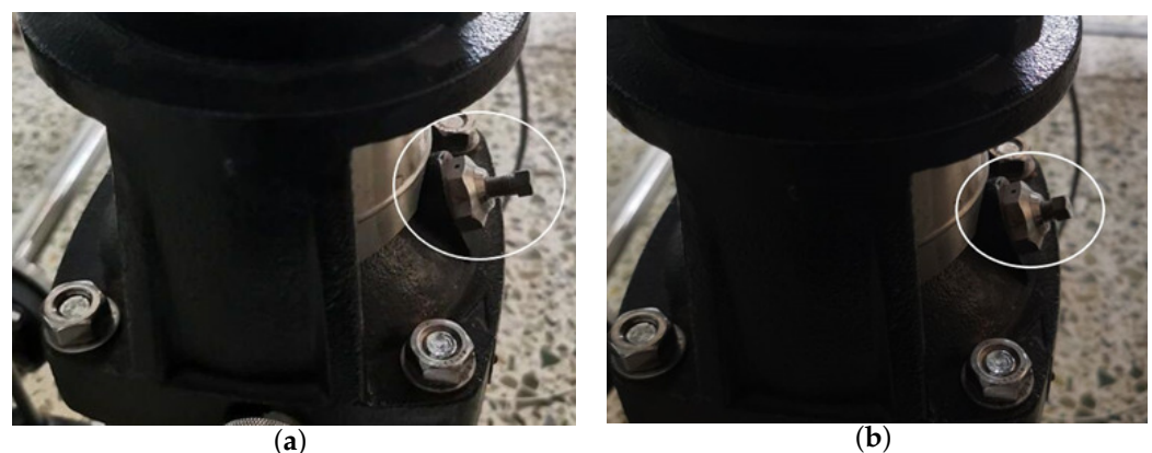
Figure 14. Air binding fault setting: (a) Exhaust screw loose, (b) Exhaust screw tightened.
