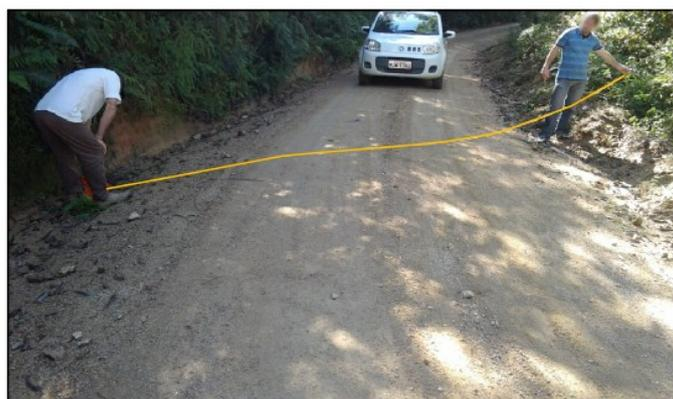
**Figure 4.** Checking the required length for a culvert.
