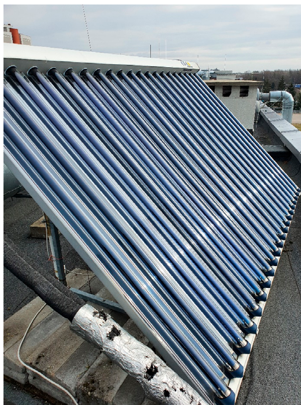
Figure 1. CPC evacuated-tube collector (own photography).
