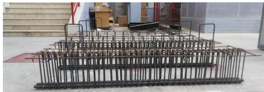
(b) Reinforcement cage
