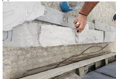
(c) Epoxy application
