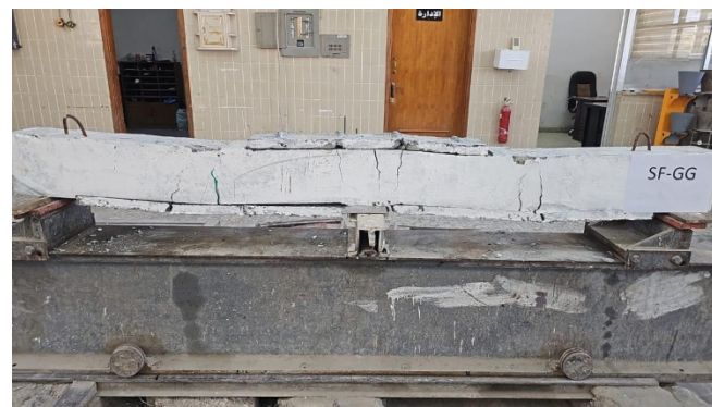
Figure 14. Failure mode and crack propagation of the SF-GG beam.
