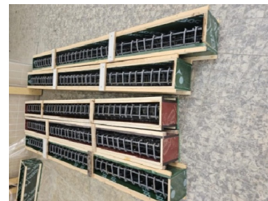
(a) Installian of steel reinforcement
