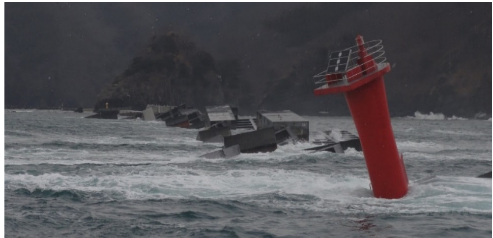
Figure 9. Breakwater damage during tsunami event.
