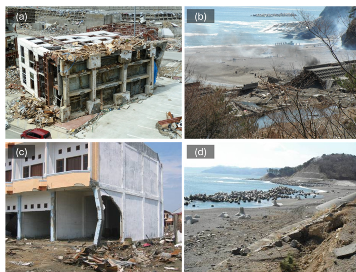
Figure 5. Various examples of infrastructure failure that occurred during past tsunami events: (a) Overturning of reinforced concrete apartment building, Onagawa, Japan, 2011, (b) shoreline protection structure failure, Tanohata, Japan, 2011, (c) Debris impact, Banda Aceh, Indonesia, 2004, (d) movement and breakage of Tetrapod armor units, Japan, 2011.
