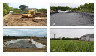
Figure 3. Stages in the construction of an evapotranspiration system: (a) excavation of basin (b) laying the impermeable membrane (c) installation of distribution layer, and (d) initial growth of the willows [29].
