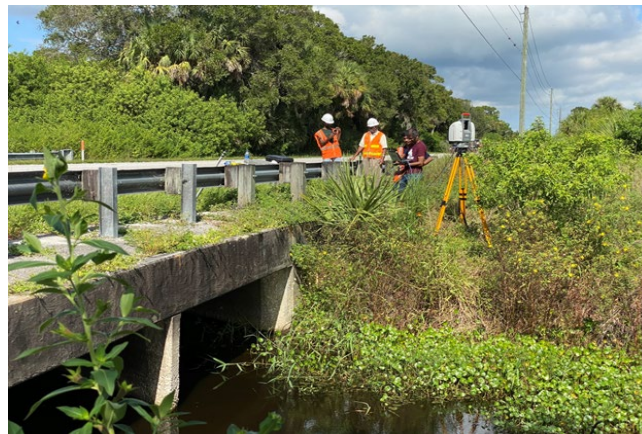
Figure 15. Leica scan station II set up for underwater scanning of SX.928 highway bridge.
