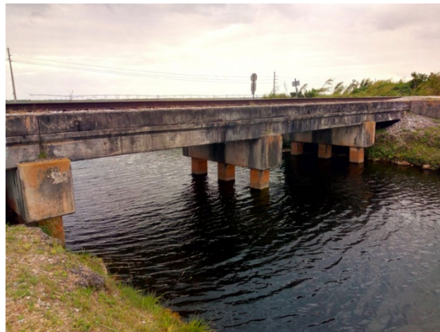
Figure 7. Pictorial view of the railroad bridge—Miami, Florida.
